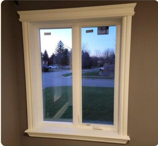
White windows, inside view
