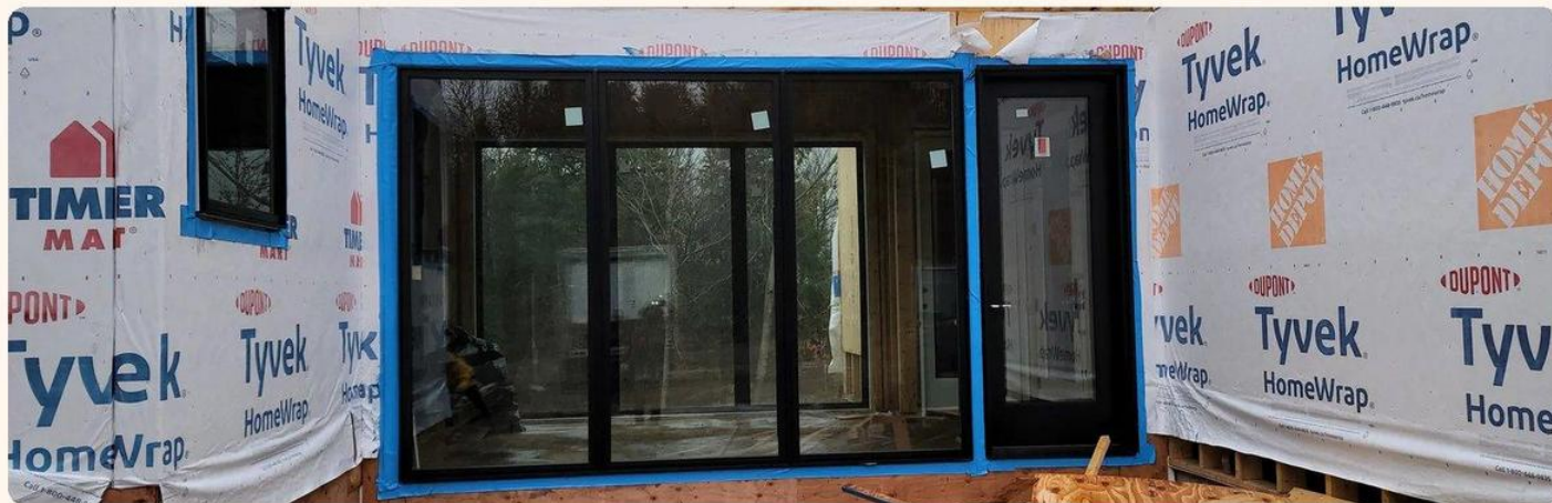
Black aluminum windows and doors going into a new build
