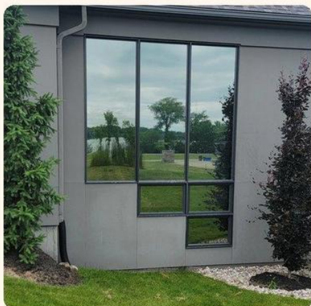
Corner windows, modern home
