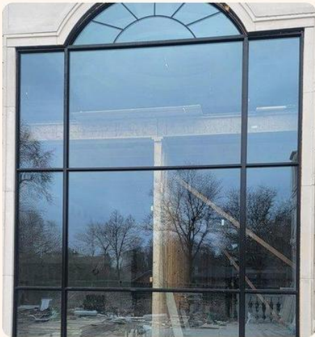
Two-storey arched glass wall
