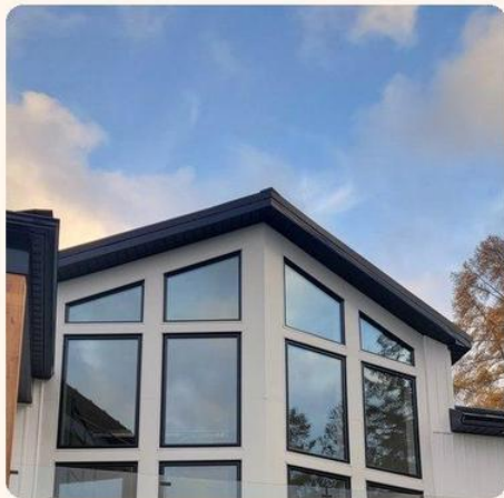
Gable window wall, new build
