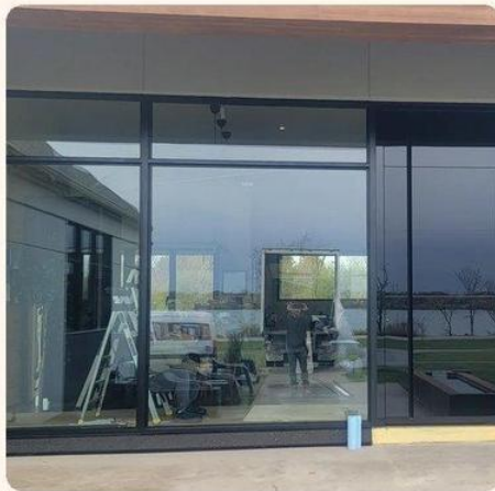
Wall of sliding glass
